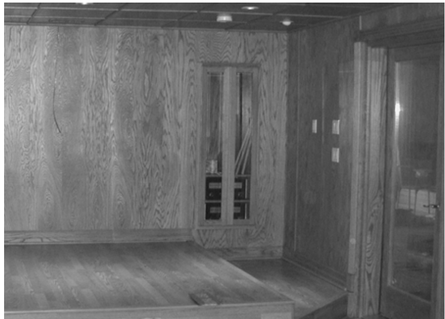
Figure 11-7. Completed back wall of HT showing door, equip- ment cabinet, riser and oak paneling. Note the sealing glass doors on the cabinet.
