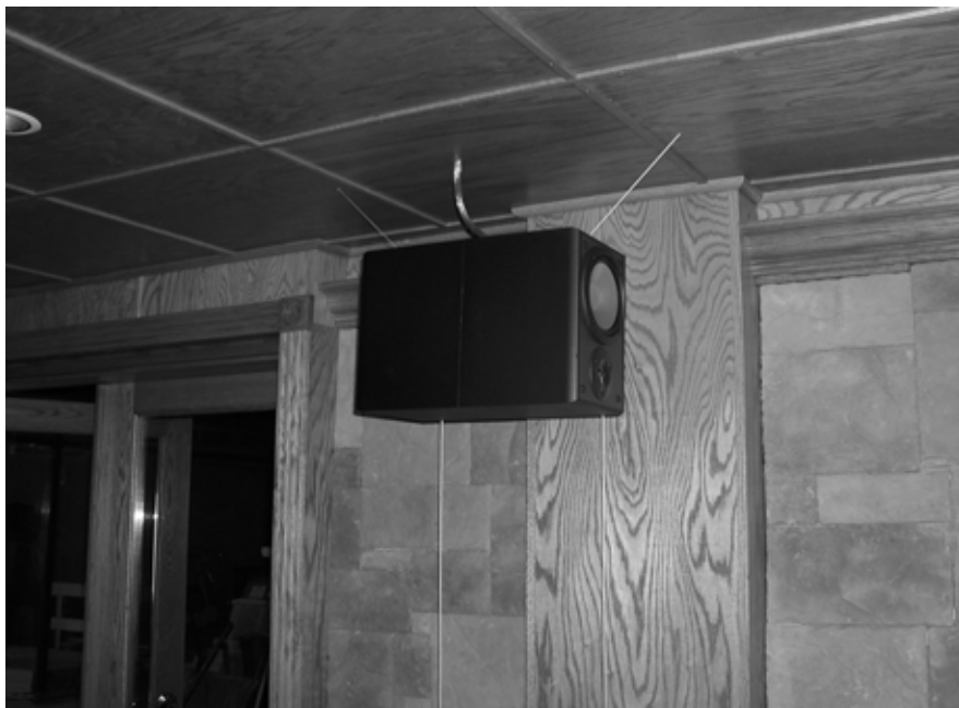
Figure 12-5. Dipole surrounds shown hanging from nylon cord for low vibration trans- mission. The door and a stone wall are visible in the background.
