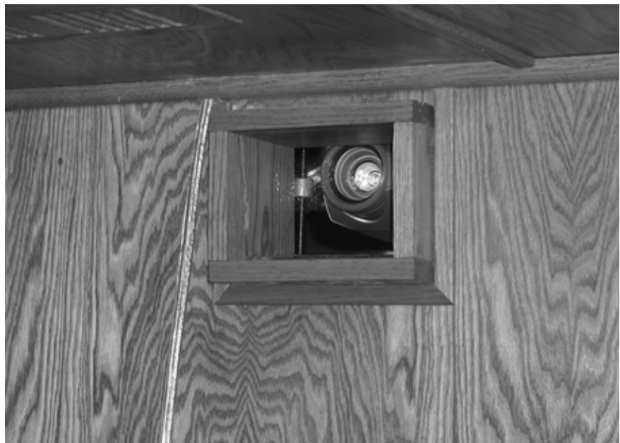
Figure 12-7. Projector mounted behind the rear wall and extending through an angled glass plate.
